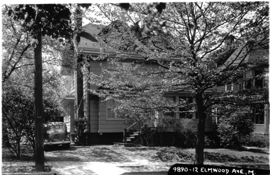
HOUSE OF REACTORS OF THE ORANGES AND MAPLEWOOD
